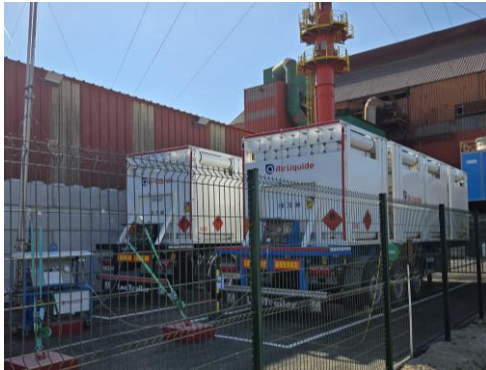
Figure 2. Hydrogen semi-trailers secured by chain-link fencing and mandatory safety clearance distances
